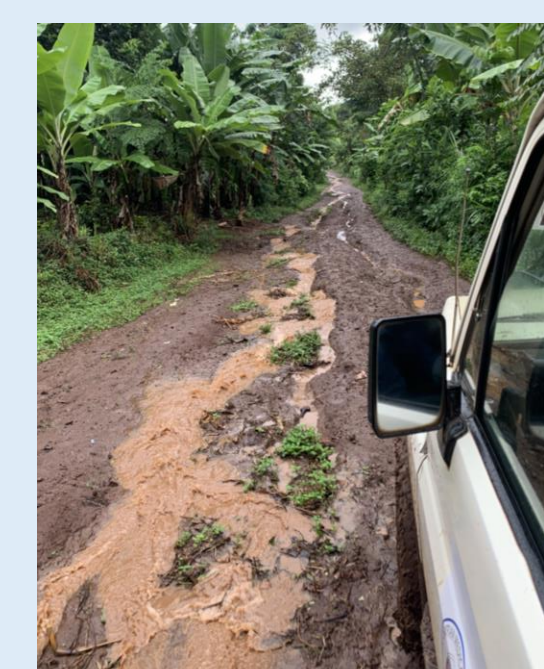
Figure 5 – Flooded road in highlands of Hai during high rainfall season
